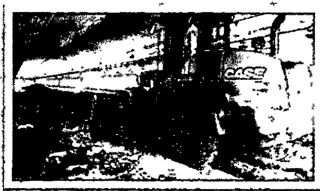
Pay loader used for clearing the base (photo by Josh Payne)
