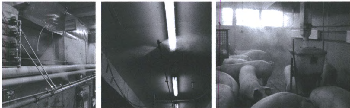
Figure 2. Air humidifying at the incoming air and indoors using separately controllable fogging lines with four and six high pressure nozzles respectively per compartment
